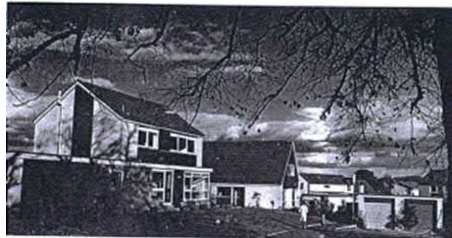
Figure 40.4 Housing at Park Way in Kildrum.
