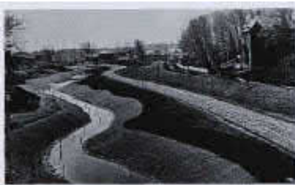
Riverway under construction, c. 1892
