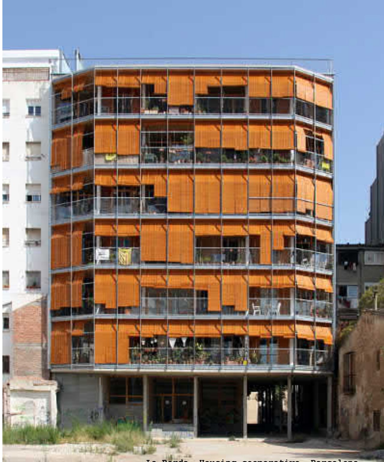
La Borda. Housing cooperative. Barcelona Lacol Arquitectura Cooperativa
