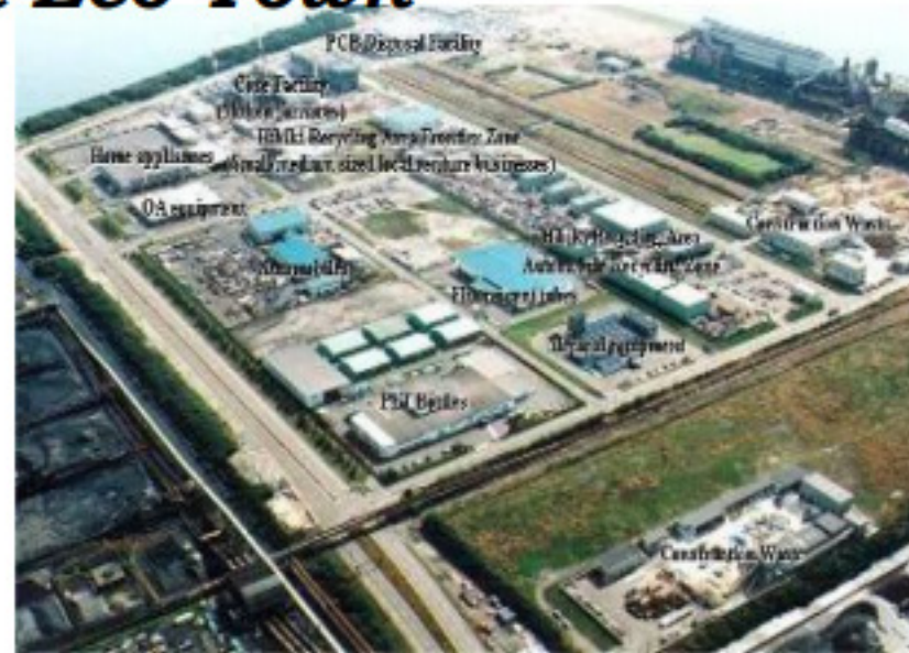
Comprehensive Eco-Industrial Complex, Hibiki Recycling Area Industrial Plants: 29
